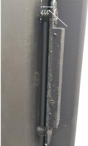
To change the pull in the door, adjust the two magnet modules.
